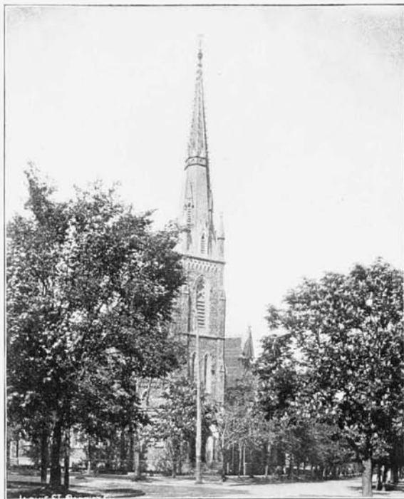
JARVIS STREET BAPTIST CHURCH.
